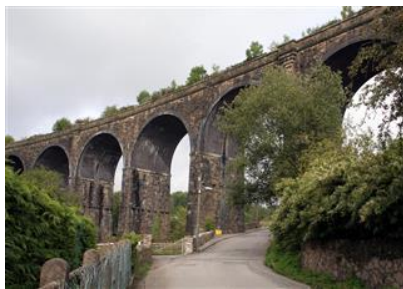
Photo of the viaduct at Garndiffaith
